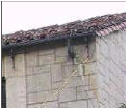
Gutter with downspout into wall
