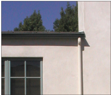
Gutter and downspout
