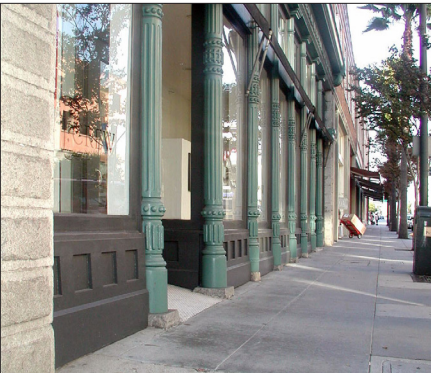
Storefront with cast iron columns
