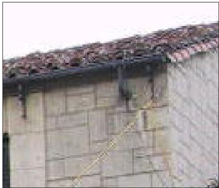
Gutter with downspout into wall
