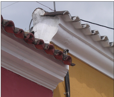
Tile on profiled parapet
