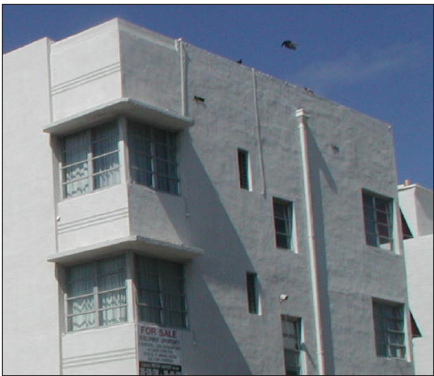
Scupper and downspout on building side
