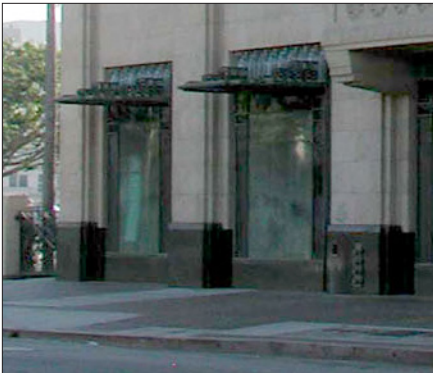
Masonry base and monolithic wall
