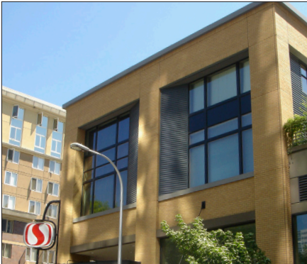
Simple brick pattern beneath parapet with cornice
