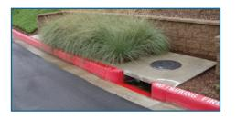
biological process working to break down and remove non-point source pollutants. The flow rate is controlled in the MWS Linear, giving the plants more contact time so that pollutants are more successfully decomposed, volatilized, and incorporated into the biomass of the Modular Wetlands'® micro/macro flora and fauna.
