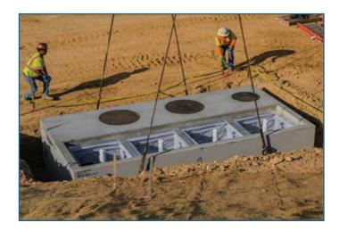
The Modular Wetlands® System Linear is simple, easy to install, and has a space-efficient design that offers lower excavation and installation costs compared to traditional tree-box type systems. The structure of the system resembles precast catch basin or utility vaults and is installed in a similar fashion.
