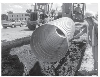
Reduced excavation because of ULTRA FLO's smaller outside diameter.
